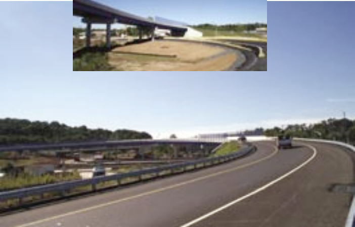
In the large photo above the new southbound “fly over” ramp rises up and over the PA 309 Expressway at Fort Washington. The inset shows the ramp passing over the partially-completed new southbound on-ramp.
