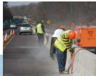
Reconstruction of the northbound side north of Highland Avenue began in 2007. Left, a crew securing a construction barrier in the northern section.
