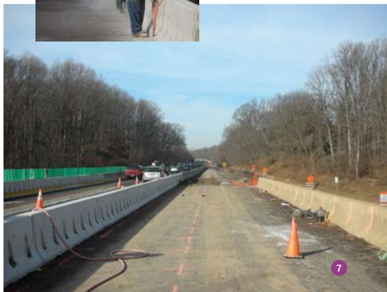
Reconstruction of the northbound side north of Highland Avenue began in 2007. Left, a crew securing a construction barrier in the northern section.
